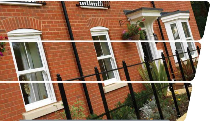
White **charisma** vertical sliding sash windows fitted onto new build property with single Georgian bar
