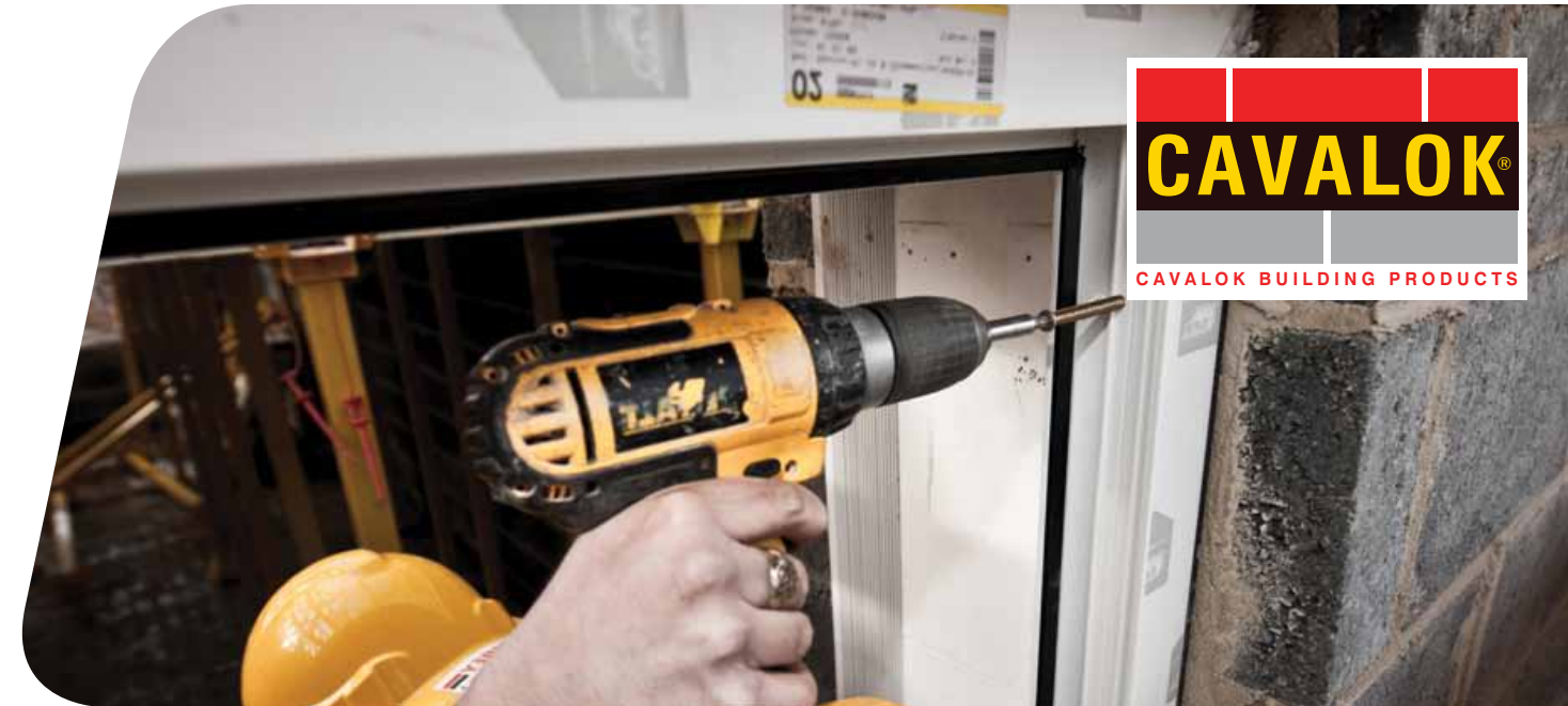
Cavalok cavity closers provide a framework for windows to be fitted from either inside or outside the building
